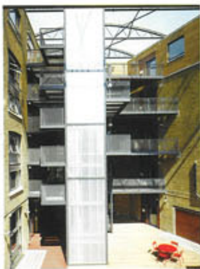
Above The ETFE roof over the courtyard springs from a timber-clad rooftop extension to the curved AM Building. Above right Photograph of the site as found and early proposals for a roofed courtyard and external circulation (ph: M&P). Below Copolastic Rodex cladding to the lift tower is back-lit at night.
