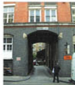
Above and right The external fabric has been extensively refurbished, with new double-glazed timber pivot windows to match the existing fenestration. The brickwork has been cleaned and repointed. The individual entrances to the old depository have been retained and certain current tenants have looked at re-using these as 'private' entrances off Clerkenwell Close.
