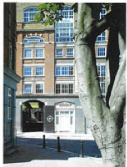
Above and right The external fabric has been extensively refurbished, with new double-glazed timber pivot windows to match the existing fenestration. The brickwork has been cleaned and repointed. The individual entrances to the old depository have been retained and certain current tenants have looked at re-using these as 'private' entrances off Clerkenwell Close.
