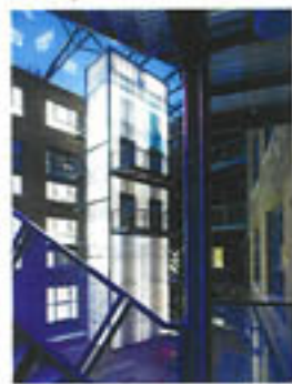
Above The ETFE roof over the courtyard springs from a timber-clad rooftop extension to the curved AM Building. Above right Photograph of the site as found and early proposals for a roofed courtyard and external circulation (ph: M&P). Below Copolastic Rodex cladding to the lift tower is back-lit at night.
